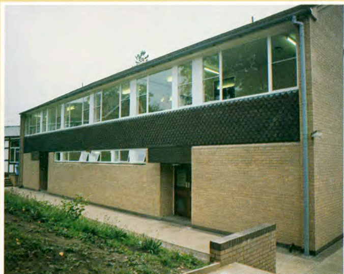
The new Hopkins Building, opened by the Duchess of Devonshire in 1983, which houses well-equipped rooms for art and crafts, mathematics and computer work.
